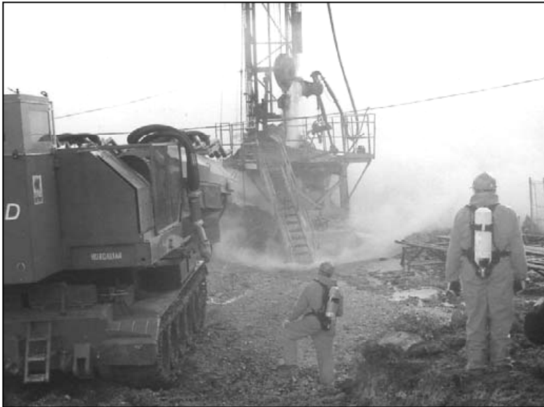
Figure C2 Melting the ice with the large capacity hot air blower
